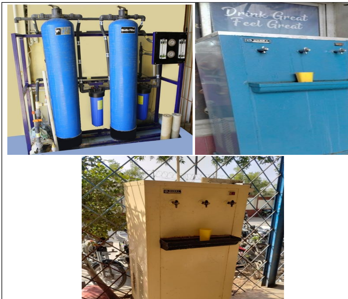
Filter Plants are place at Main Campus that use to remove impurities from water
